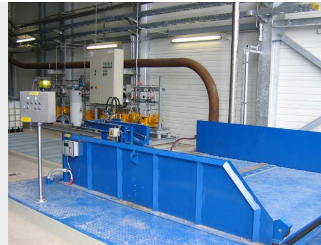
Above: Automatically controlled flaps are an important feature of receiving bunkers. Putzmeister offers a range of different variants.
